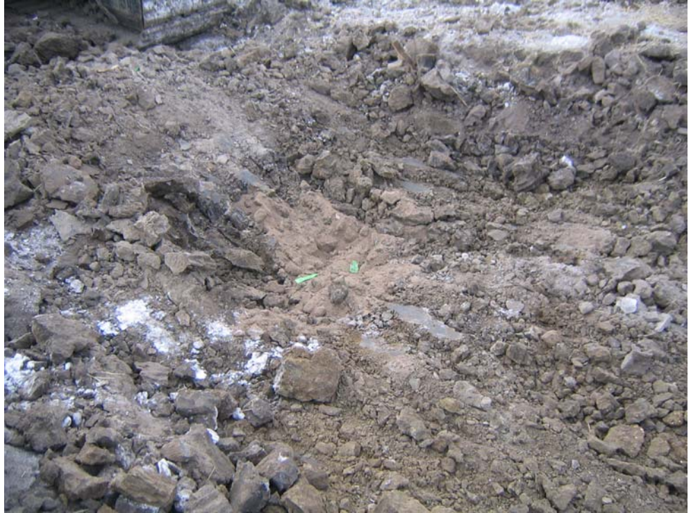
This photo provides a clear view of the exposed green sections of the Line Alert panel following a pass of the bucket.
