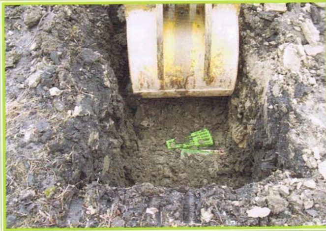
At left: Excavator encountering the panel. Above: Clear reading of the depth from the line – 32 inches.
