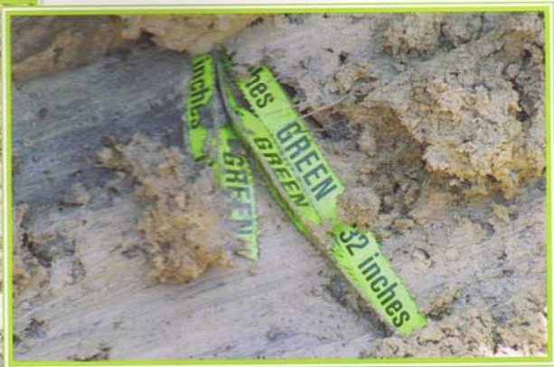
At left: Excavator encountering the panel. Above: Clear reading of the depth from the line – 32 inches.
